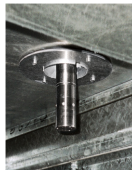
Typical sensor installation
